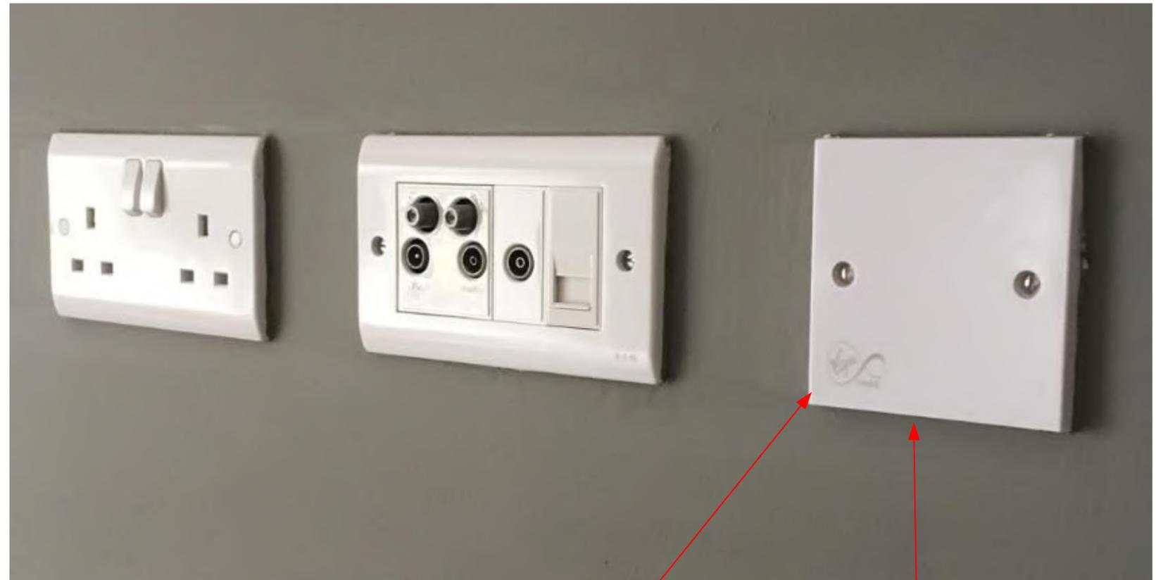
When using Media plates (see also drawing VMTD0048a) then please ensure that Virgin Media wiring is segregated from other operators. This ensures enough space within the back box to work the cabling and insert any splitters/isolators.
