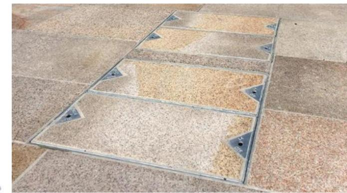
Recessed covers are tested (unfilled) to the B125 load classification and can be filled with any material to suit the surrounding area.
