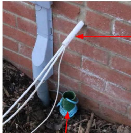
uPVC duct must be cut back before pulling cables externally, this prevents damage to cable while trying to tidy at 2<sup>nd</sup> fix.
