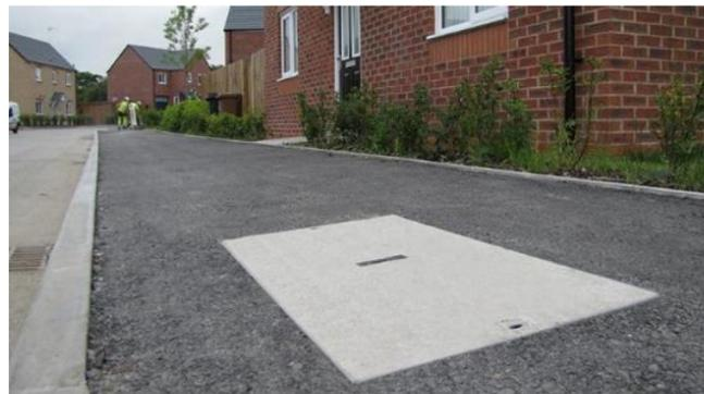
Cubis AX-S™ Concrete Infill covers are the sole approved footway cover used by Virgin Media.
